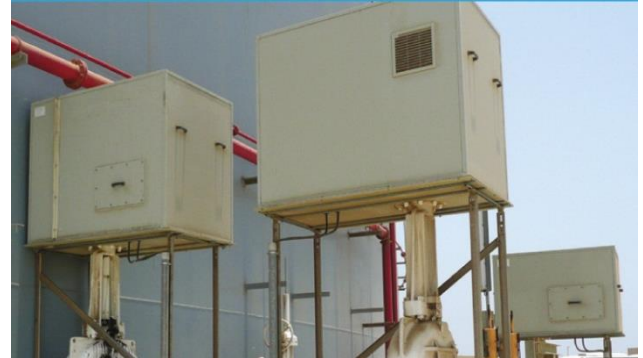
Fire Shelter for Valve- Actuator
