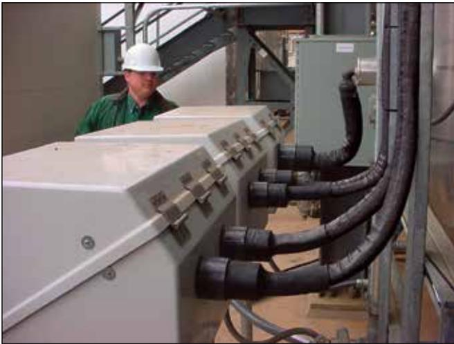
Small diameter lines are heated for many reasons including freeze protection (winterization), reduced viscosity, and keeping gas samples above their dew point. These can be critical for process accuracy, emissions compliance, and even plant operation.
